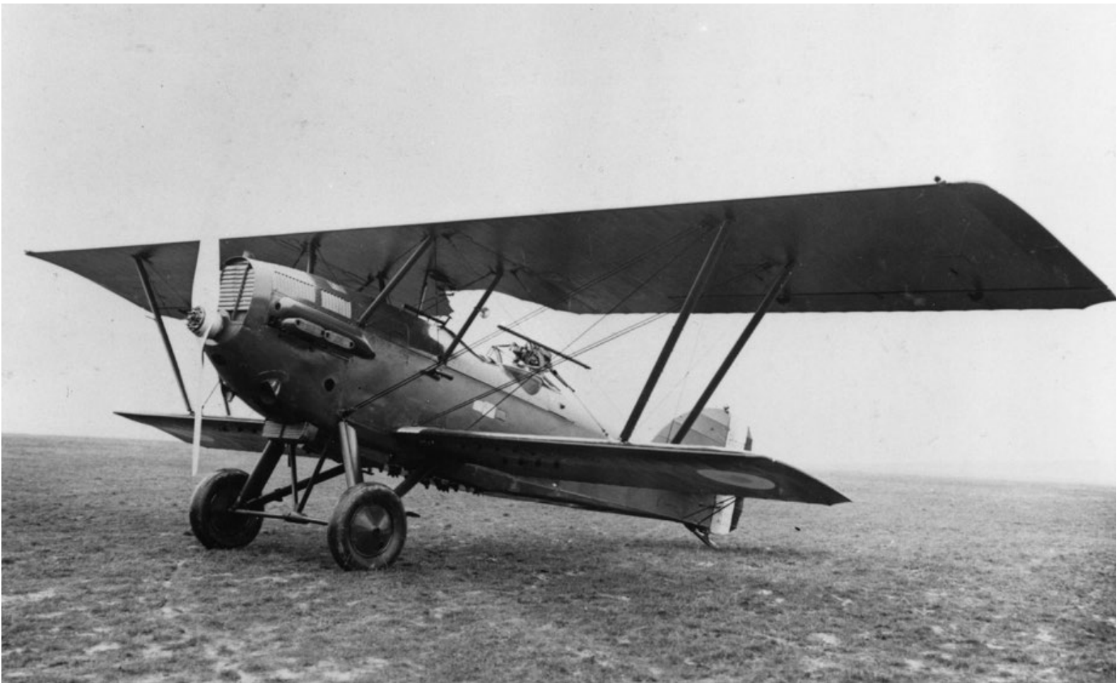
1925 - COMMISSIONING OF THE POTEZ 25 The Potez 25 biplane came in two versions: for civil and military use. It was the most frequently manufactured French aircraft of its time with around 4,000 planes being built and also exported to 22 countries.
