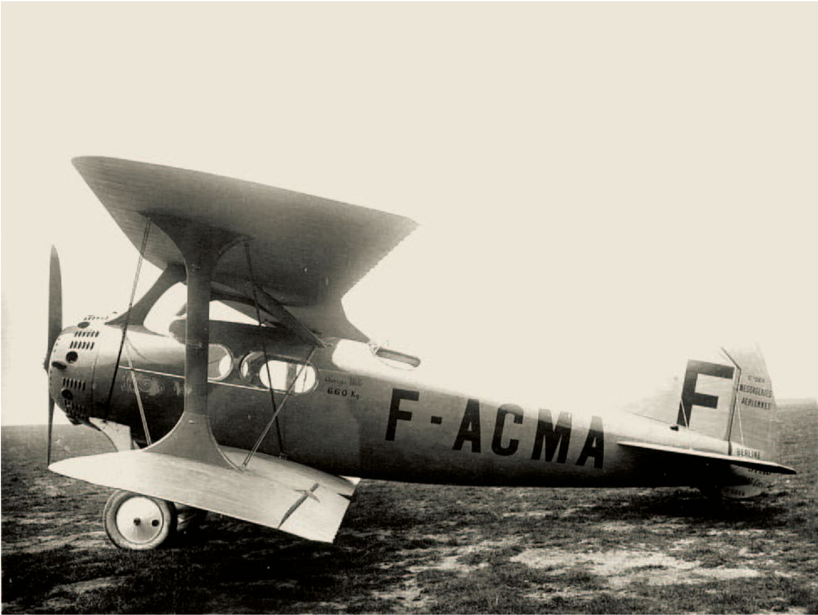
JUNE 16, 1921 - MAIDEN FLIGHT OF THE SPAD S.46 BERLINE The SPAD S.46 Berline was a further development of the SPAD S.33. It was able to transport five passengers, four seated in wicker chairs in the closed cabin and one in the cockpit next to the pilot.
